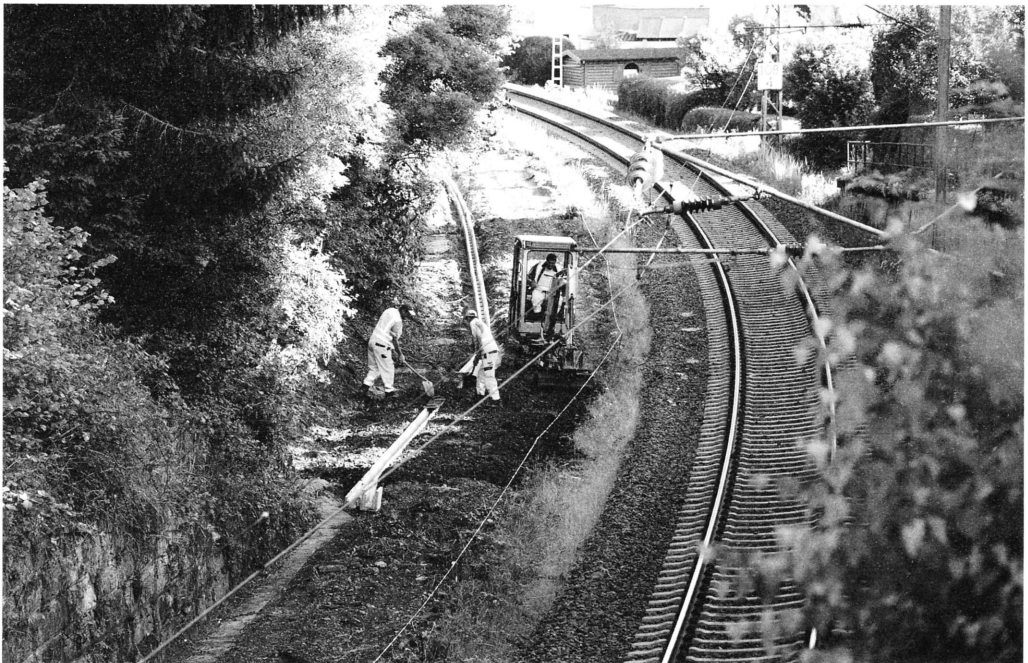
Abb. 7: Kabelkanalbau. Construction of cable pits.
